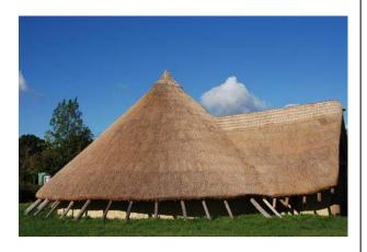
Our house was built in stages: first the main pillars were erected, and the horizontal beams attached with wooden pegs. The outer walls were constructed from hazel wattle fencing which was then covered on both sides with 23 tonnes of daub, a mix of clay, sand and straw. The rafters and roof battens were added, with 2 miles of rope used to lash it all, and the roof was then professionally thatched with water reed. Materials such as the clay and hazel came from the local countryside.
