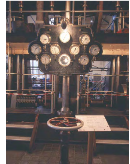
Langford steam pumps
