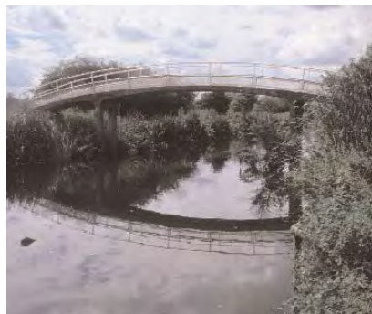
Ulting Wick Bridge
